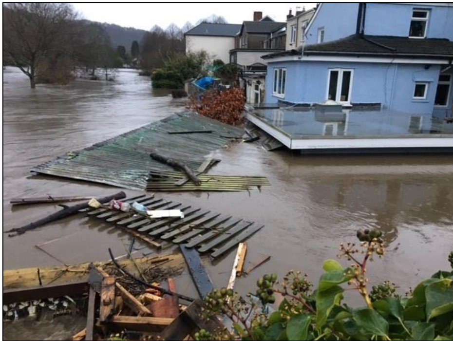
Figure 5: Image showing the overtopping of the River Taf to the rear of Cardiff Road which submerged the rear gardens and ground floor of several properties during Storm Dennis (image provided by resident)
